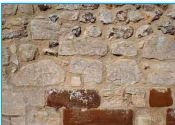
Swanage brick produced using local Wealdon clay, and a wall containing an unusual mix of local flint, limestone and heathstone.
